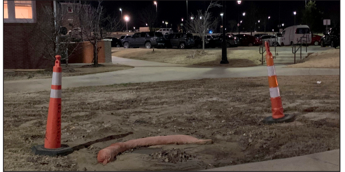
The remainder of the construction on the burst pipe
