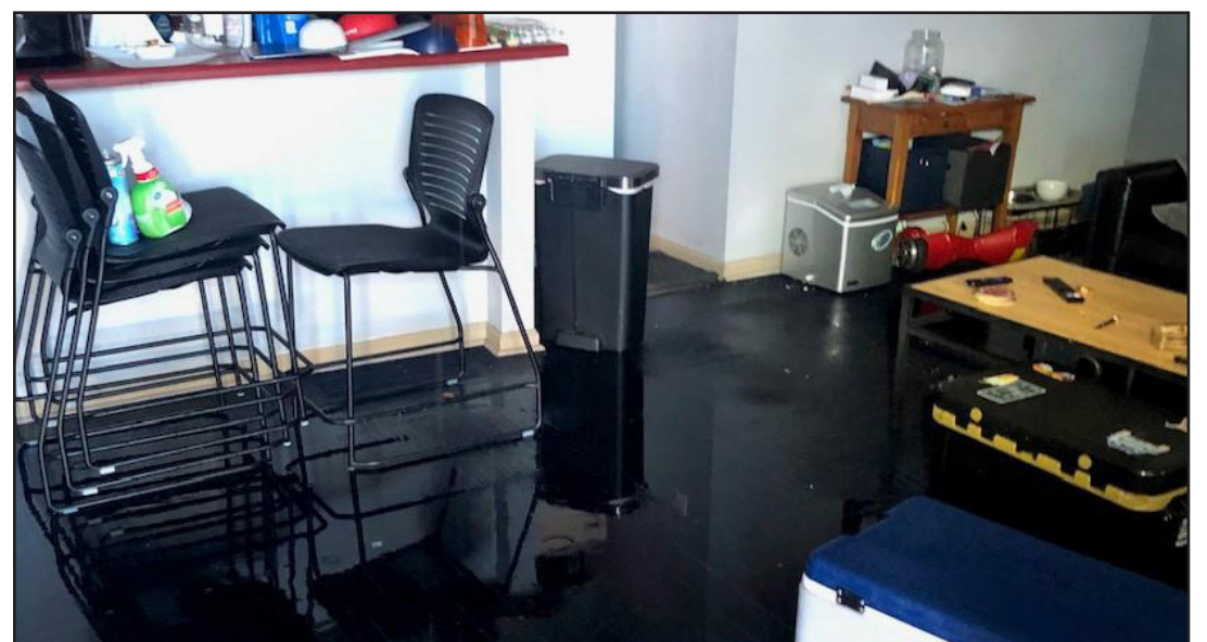
The flooding in Nicholas Palacios’ Collegiate Park Building 5 apartment.
