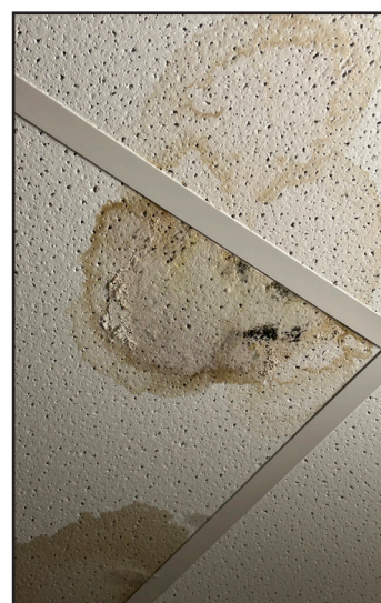
Mold growing on ceiling panels in Zoe Mathes', a junior strategic communications major from Forrest City, Arkansas, dorm. The mold was caused by a water leak and was removed by maintenance.
