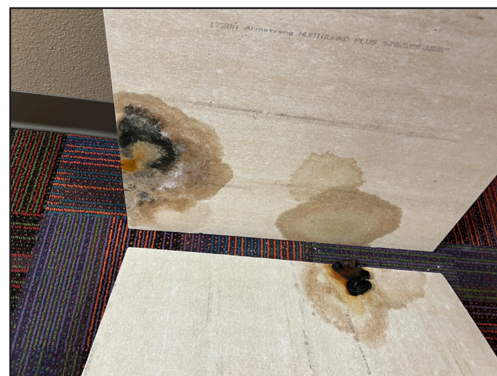
Mold growing on ceiling panels in Zoe Mathes', a junior strategic communications major from Forrest City, Arkansas, dorm. The mold was caused by a water leak and was removed by maintenance.
